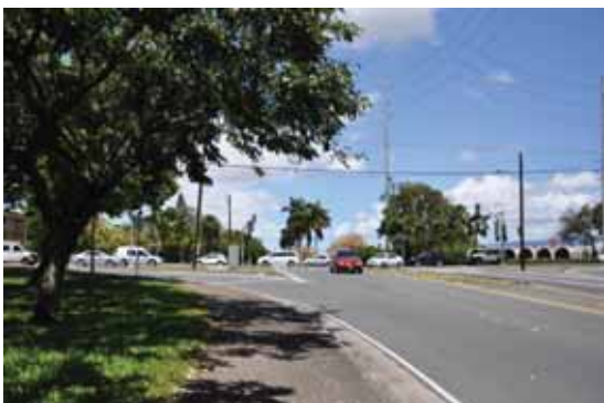
Photo 3-14: Existing sidewalk adjacent to Pearl Harbor station along Radford Drive near intersection with Kamehameha Highway
