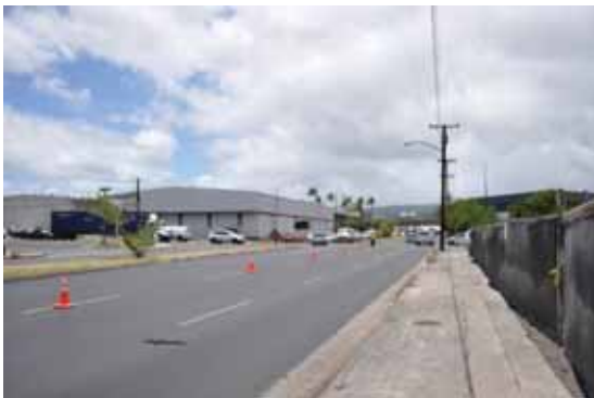
Photo 3-23: Lagoon Drive station site to the right looking toward Ualena Street intersection (looking mauka)
