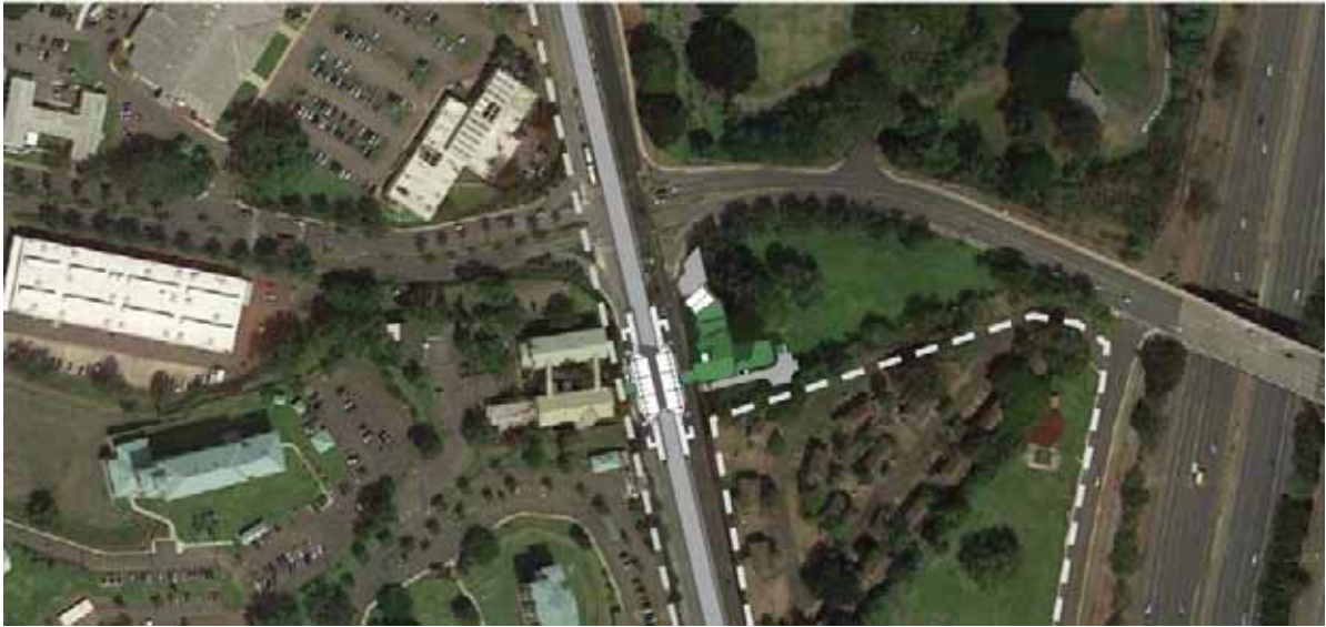
Photo 3-2: Pearl Harbor station site, showing the station facilities within the existing open space area and surrounding Navy facilities
