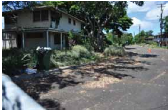
Photo 3-10: Example of underutilized land - unoccupied homes in the Little Makalapa housing area
