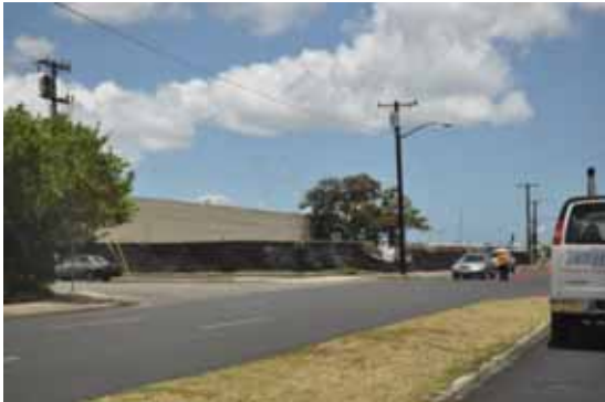
Photo 3-22: Lagoon Drive station site and looking toward Waiwai Loop
