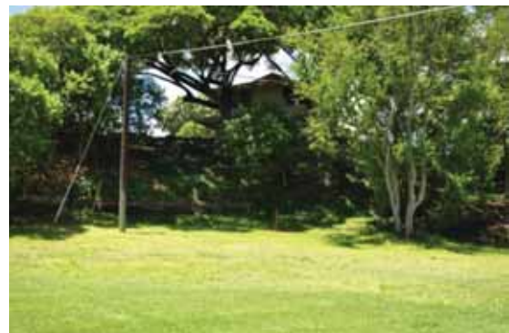
Photo 3-1: Unoccupied and dilapidated Little Makalapa Navy home above Pearl Harbor station site
