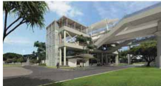
Photo 3-17: Airport station entrance and pedestrian walkway to the parking garage and elevated rail system
