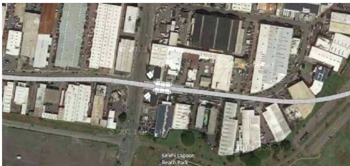
Photo 3-21: Lagoon Drive station site, showing the station facilities within the existing open space area
